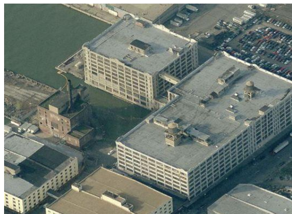
Figure 58: A M Cosmetics Building site photo
