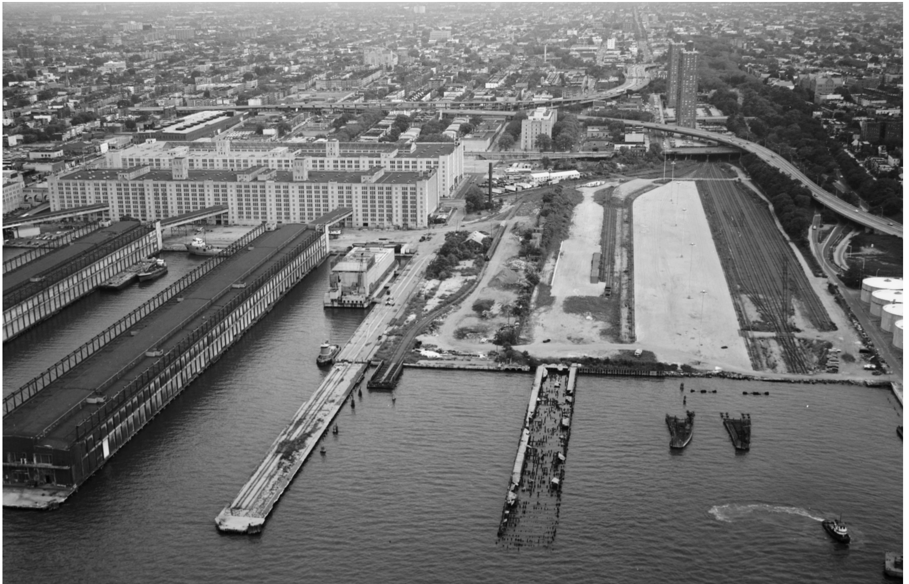
Figure 1: Historic image of the Brooklyn Army Terminal
