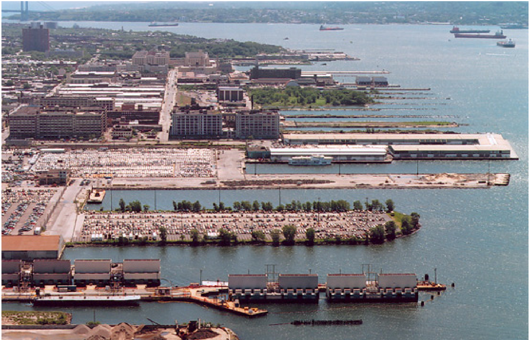
Figure 78: South Brooklyn Marine Terminal
