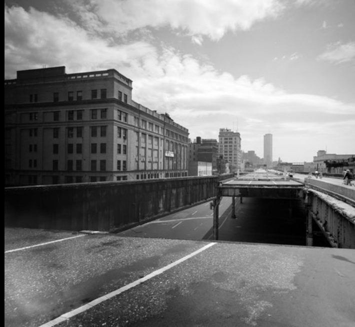
The elevated West Side Highway was torn down in 1989. Credit: New York Public Library.
