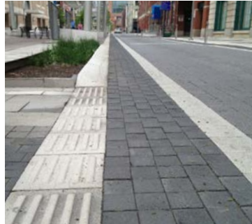
Concrete Unit Pavers Indianapolis, IN
