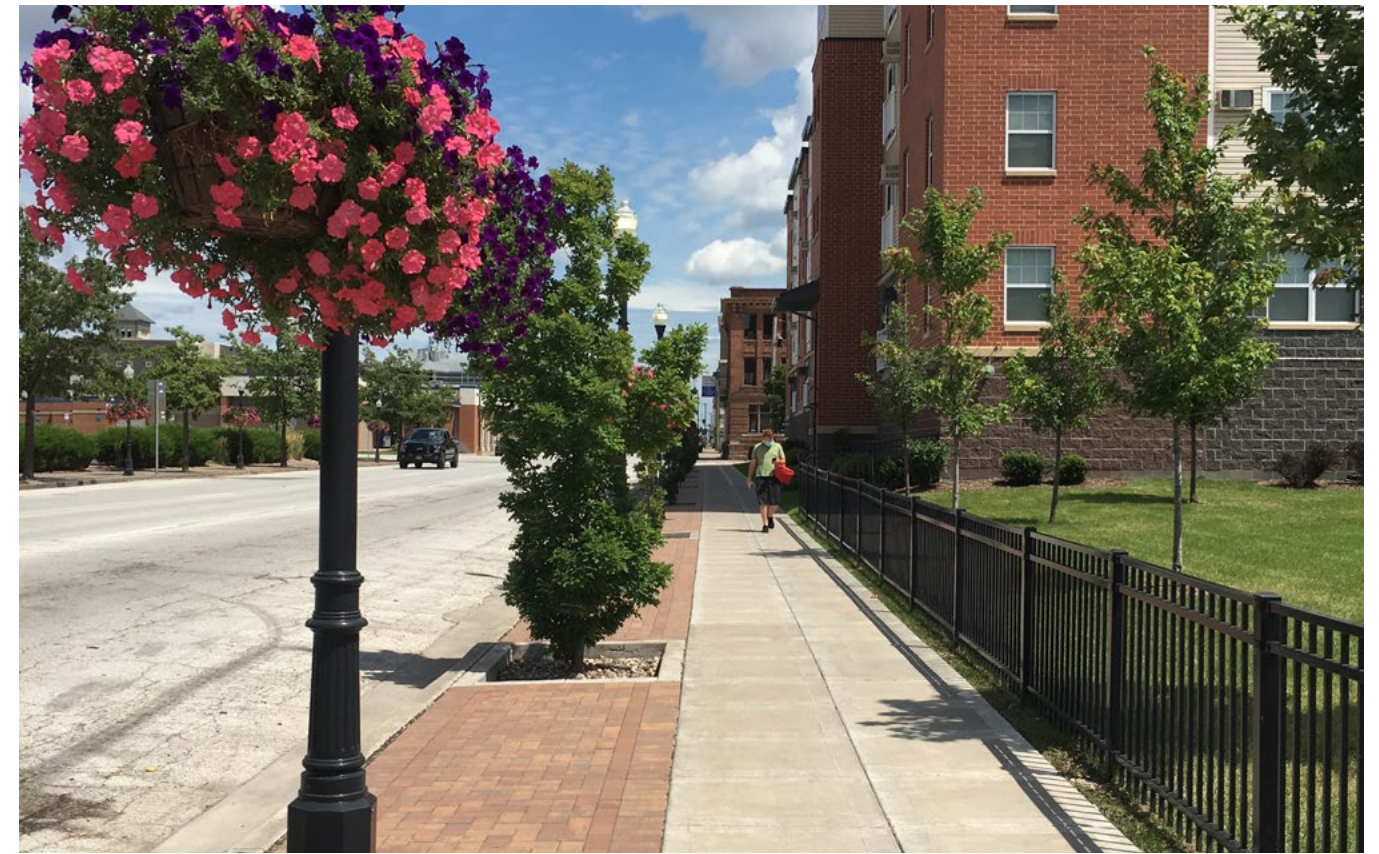
Newly constructed streetscape on 3rd Street
