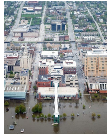
Flooding of Downtown Davenport, 2019
