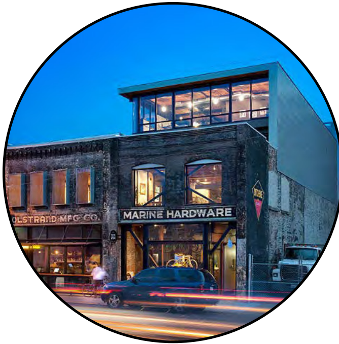
LIVE/WORK Kolstrand Building Ballard, Washington
