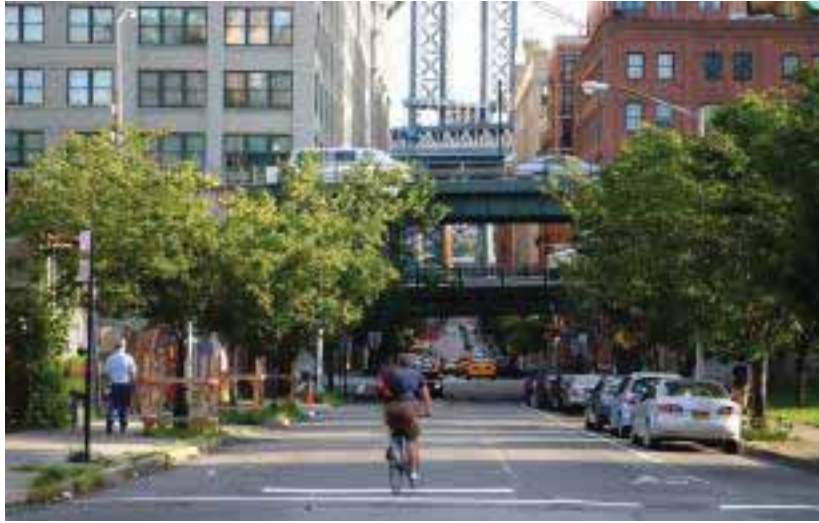
View of the Manhattan Bridge in DUMBO.
