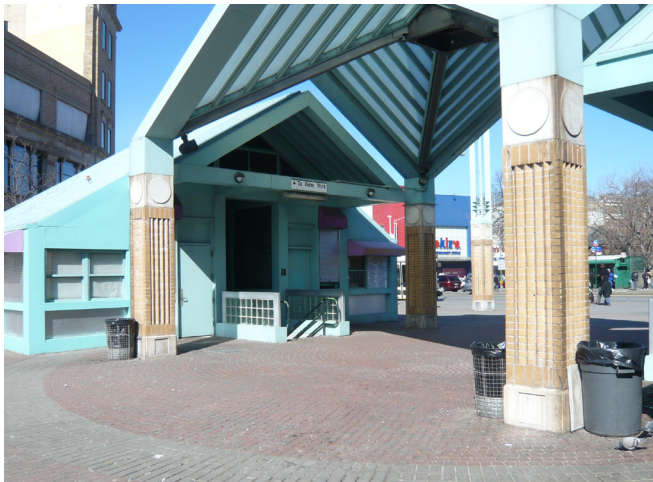
MNR station stair entry at Plaza
