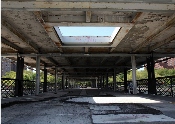
Existing roof at Pier 107 Anton Brookes, Courtesy of CIVITAS
