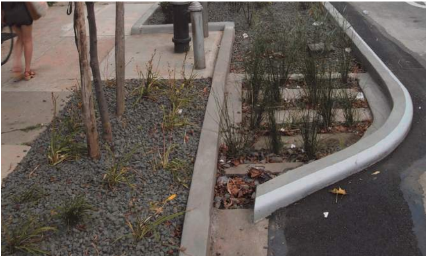
NYC DEP Bioswale
