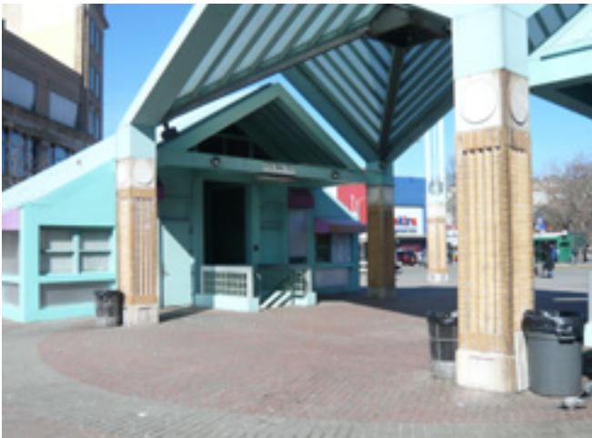
MNR station stair entry at Plaza
