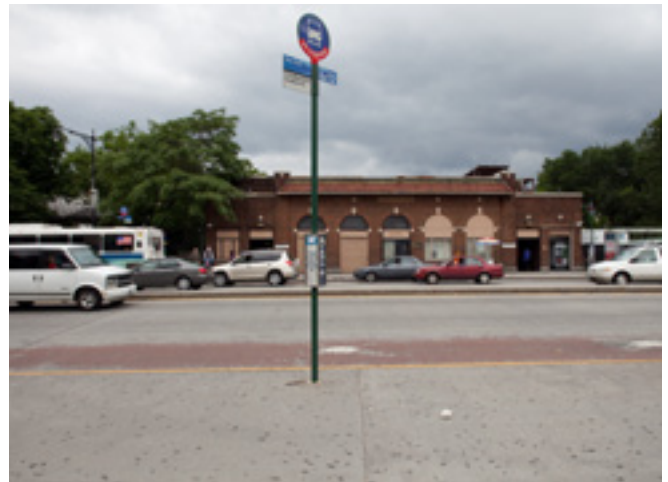
View from south side of Fordham Rd to historic Fordham MNR Station
