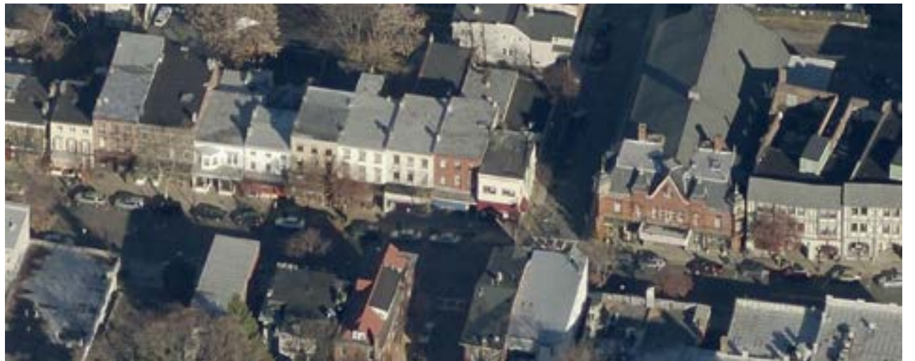
Town center as prototypical site: Aerial view of Tarrytown center
